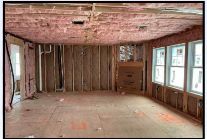
1st Floor Ceiling
